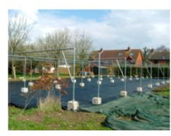
The tunnel is constructed totally above ground using a steel framework anchored into concrete blocks. The framework is integral to the bench design, which will also help to anchor the construction once loaded with plants.
